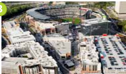
The Battery, Cobb County, GA 4.2 M SF | 700K Under Con. | 1.7% Vacancy
